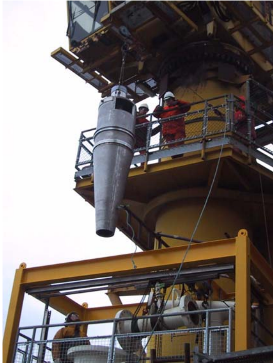
Fig. 5 – Shell Leman Delta WDC insert being installed
